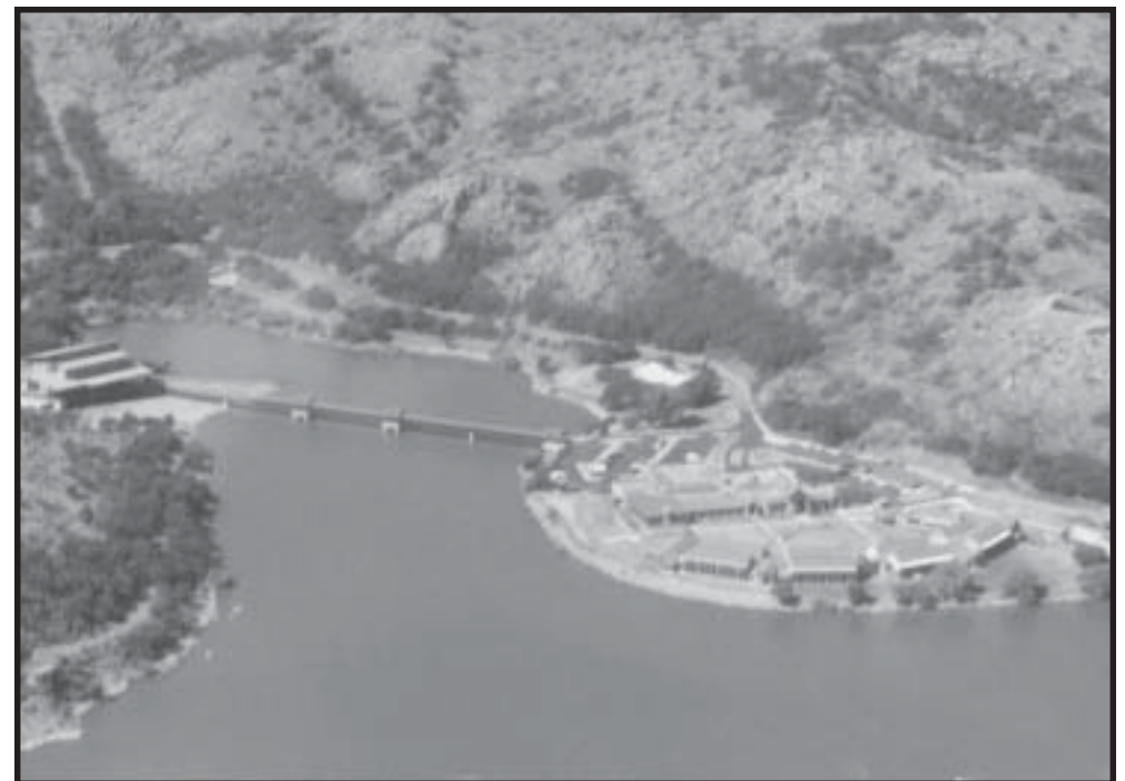
An aerial view of the Quartz Mountain Lodge complex. On the right, the lodge and four buildings with guest rooms surround a lovely central courtyard. On the left across the bridge is the Oklahoma Art Institute.
