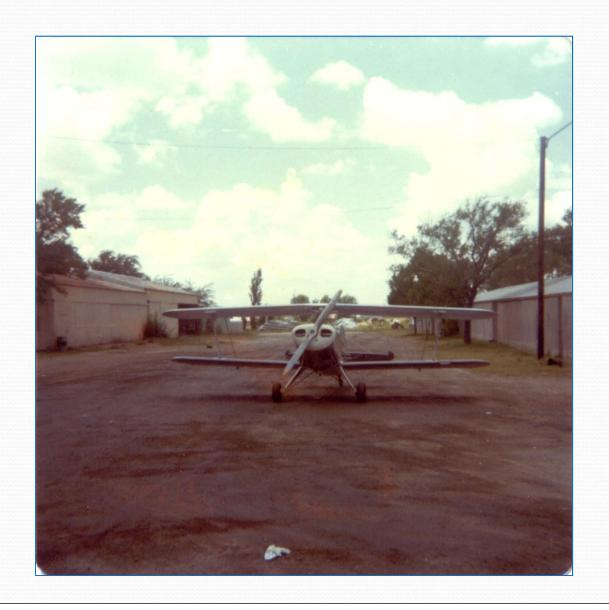
First takeoff- July 10, 1976! Lots of power, bring the tail up, keep it straight with right rudder, and rotate at about 65 mph! Fantastic climb! Lower the nose a little for visibility and climb, circle the airport at up to about 5000 feet, check things out. It all was working great engine running perfectly, airplane in trim, and controls very effective.
